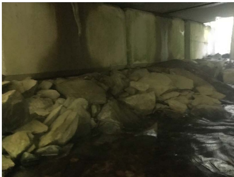
Left Bank Abutment when facing downstream
