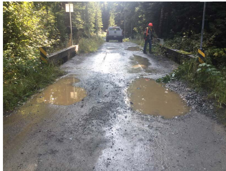
Right Bank Abutment when facing downstream
