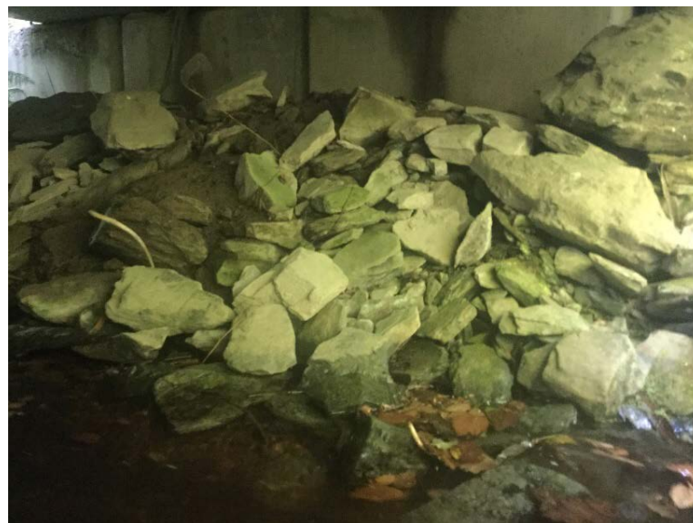
Right Bank Abutment when facing downstream
